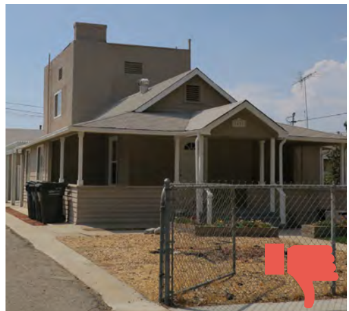
Avoid additions that are not compatible with the scale and style of the building.
