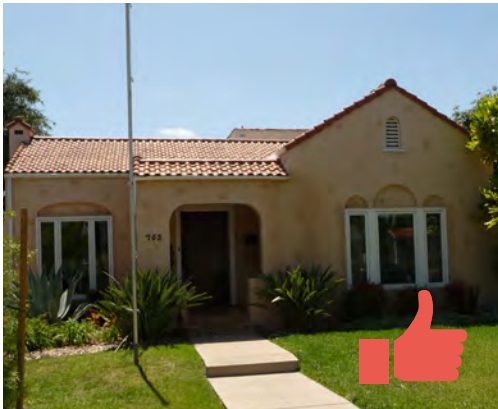
An example of a minimally visible, appropriate roof addition at the rear of a building.
