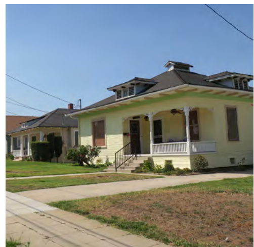
A row of Victorian style cottages.
