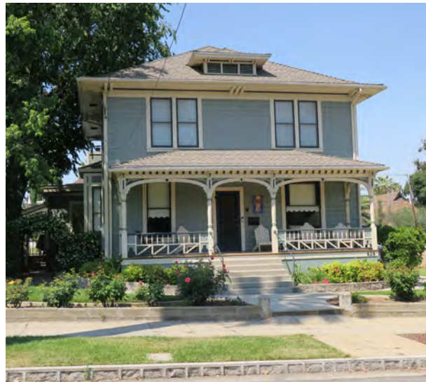
An example of a two-story, single family house within the historic district.
