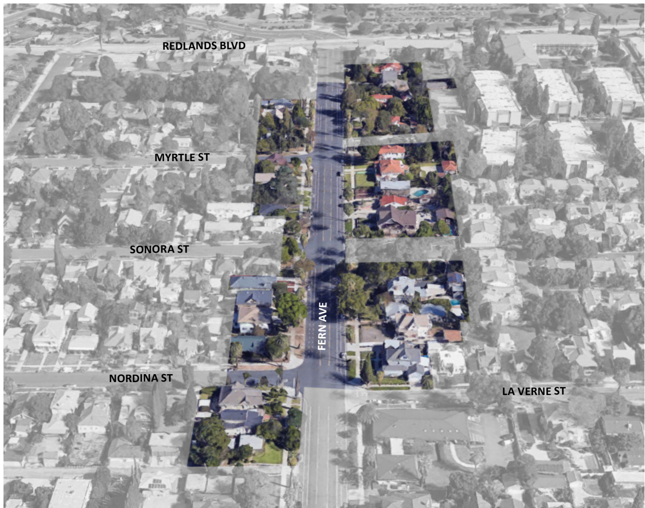
Aerial view of East Fern Ave Historic & Scenic District.
