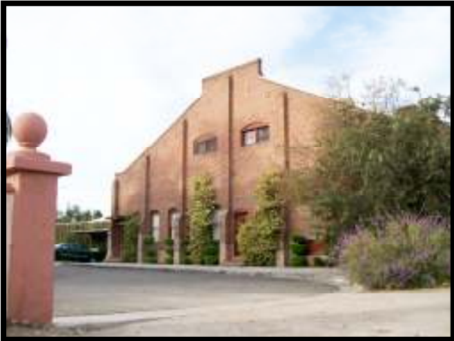
Former packing house used as a reception hall.
