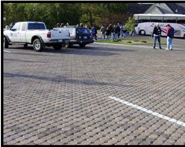
Permeable paving used for parking stalls.
