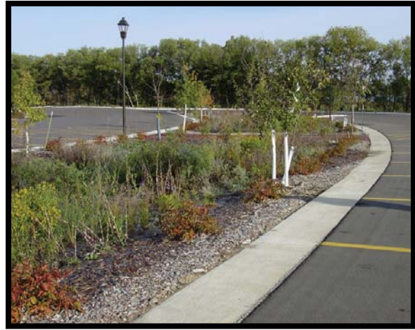
Vegetated swale with a zero-curb used as a parking lot planter.
