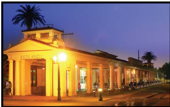
New glass panels enclose a portion of the original colonnade
