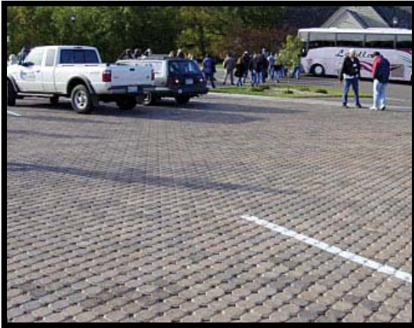
Permeable paving used for parking stalls.
