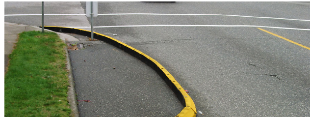
Temporary Curb Extension
