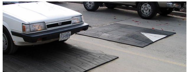
Temporary Speed Cushion
