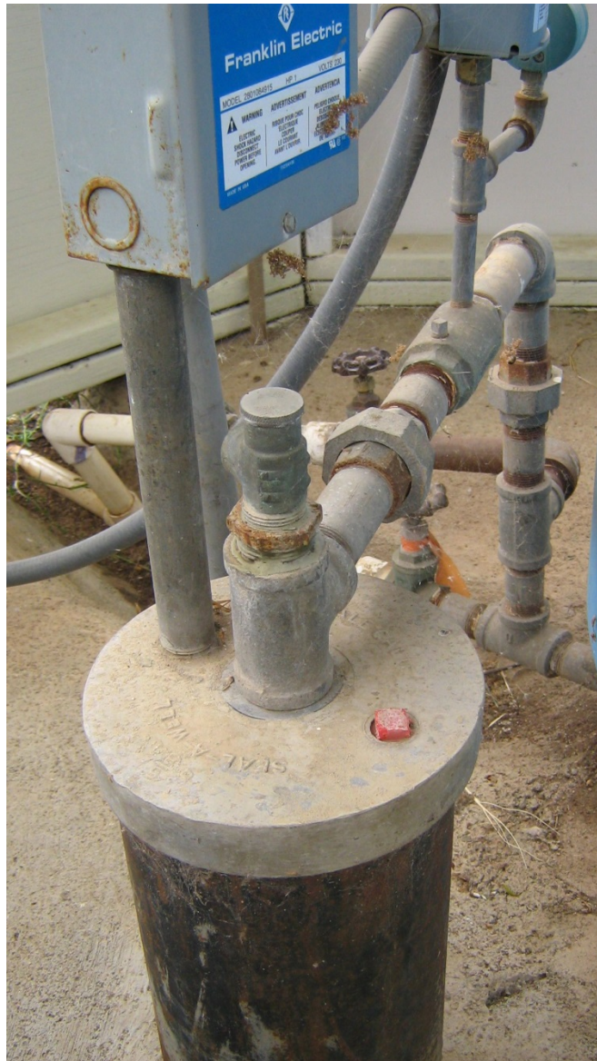
Figure 9. Photo: A domestic well showing the well casing, cover, and conveyance system.
