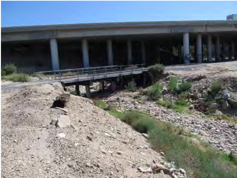
Photo 4. Looking northeast at a railroad bridge over Mill Creek Zanja just west of the I-10 overpass.
