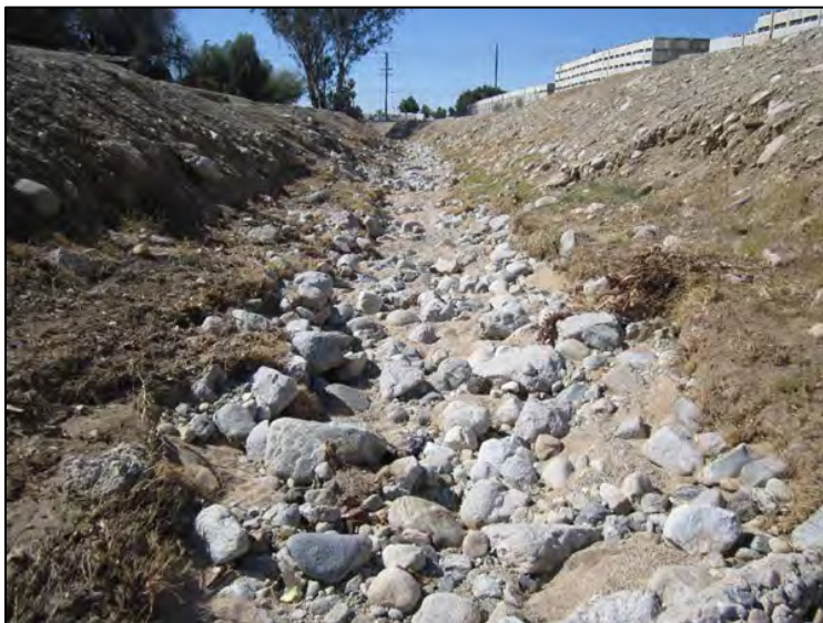
Photo 2 - Mill Creek Zanja between 9 th Street and Church Street facing west.
