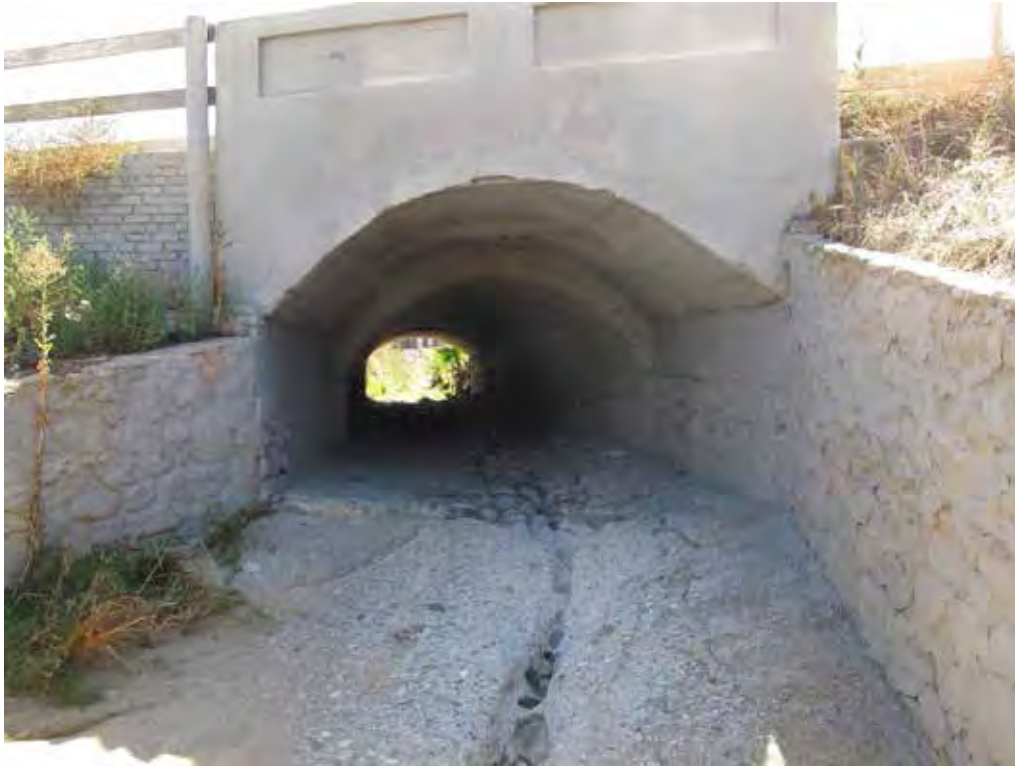
Photo 3. Looking east at Mill Creek Zanja where it crosses below Church Street.
