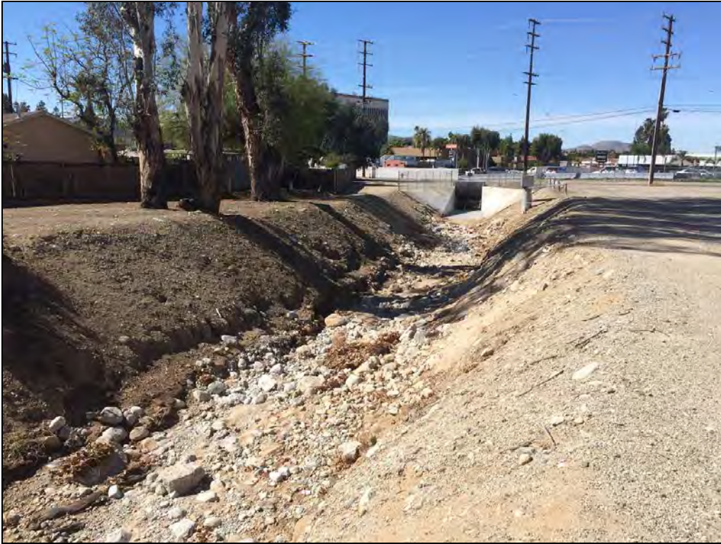
Photo 3: Zanja channel east of 9 th Street; facing southwest.
