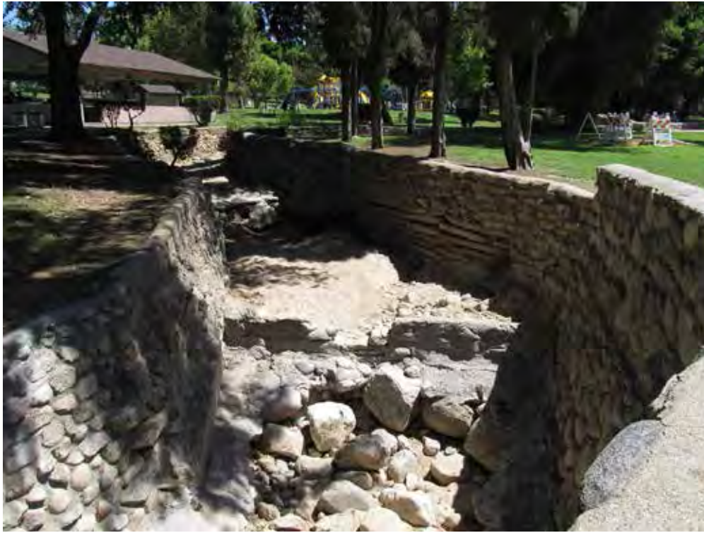
Photo 7. Looking northeast at Mill Creek Zanja as it traverses Sylvan Park.
