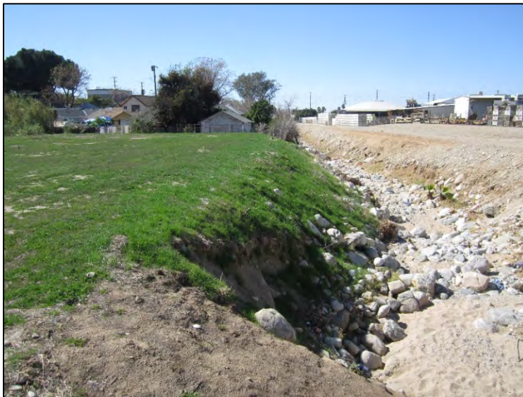
Photo 1 - Mill Creek Zanja between 9 th Street and Church Street facing west.
