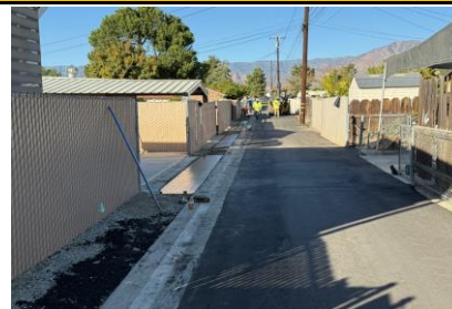
Proposed drive approach connected to the V-gutter
