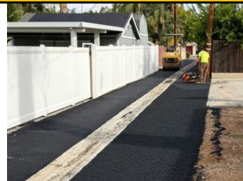
CONTRACTOR PAVING ALLEY WEST OF NORWOOD ST
