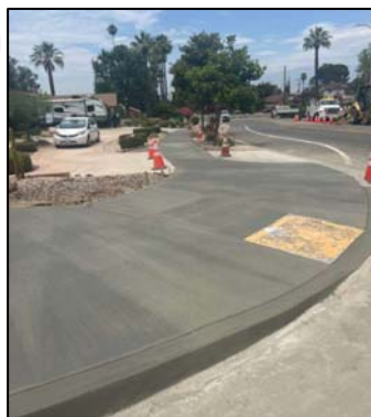
New ADA Ramp at Lakeside Avenue
