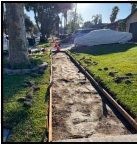
Grading, setting forms, and placing concrete on Raemee Avenue
