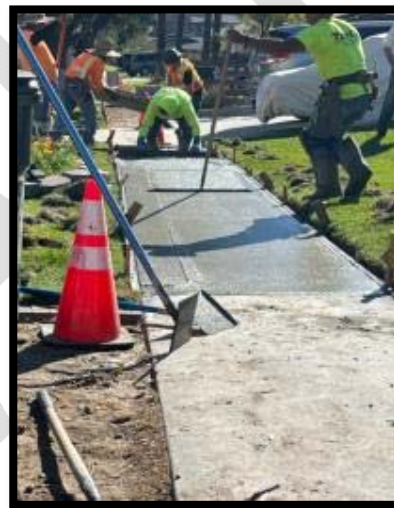
Grading, setting forms, and placing concrete on Raemee Avenue
