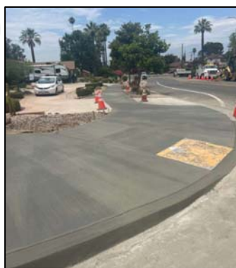
New ADA Ramp at Lakeside Avenue
