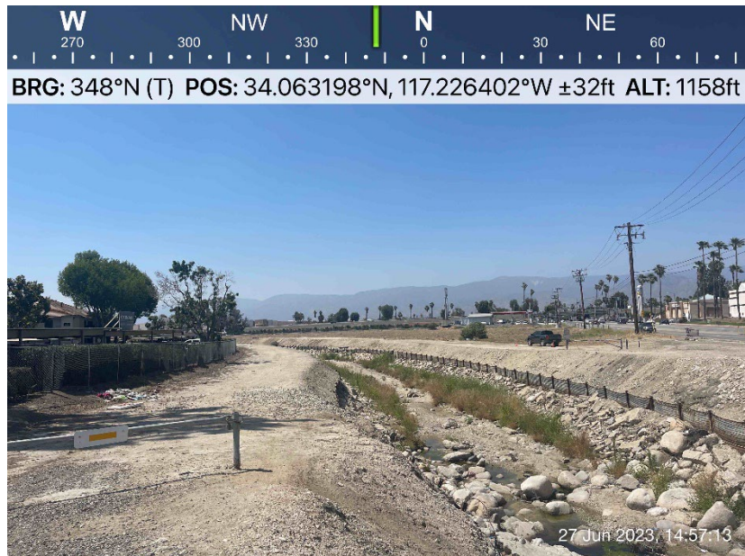
Photo Point 6. OHWM visible at toe of slope near vegetation line. TOB visible at Barrier fence.
