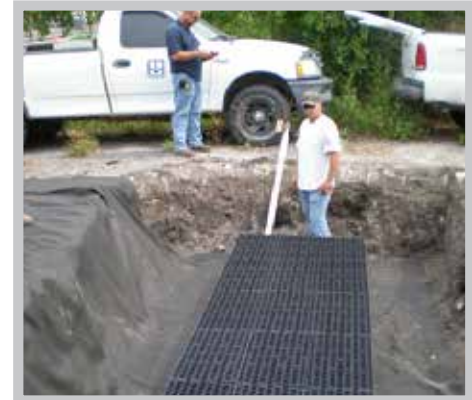
R-Tank field testing.
