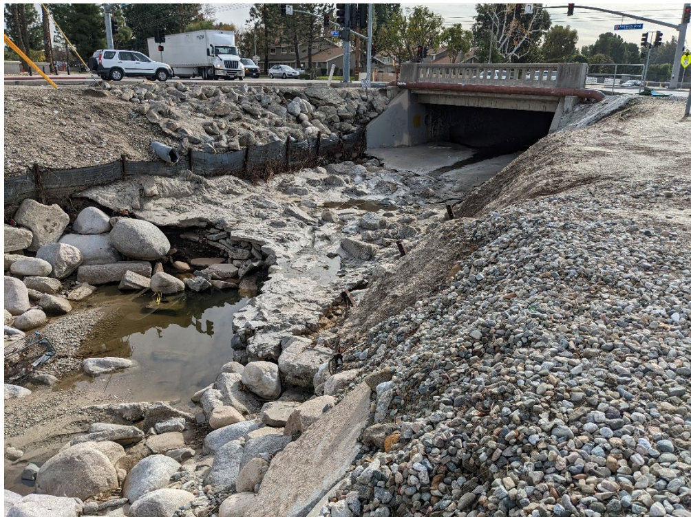
Figure 9. Overview of Mission Creek Channel and Redlands Boulevard culvert, looking southeast.
