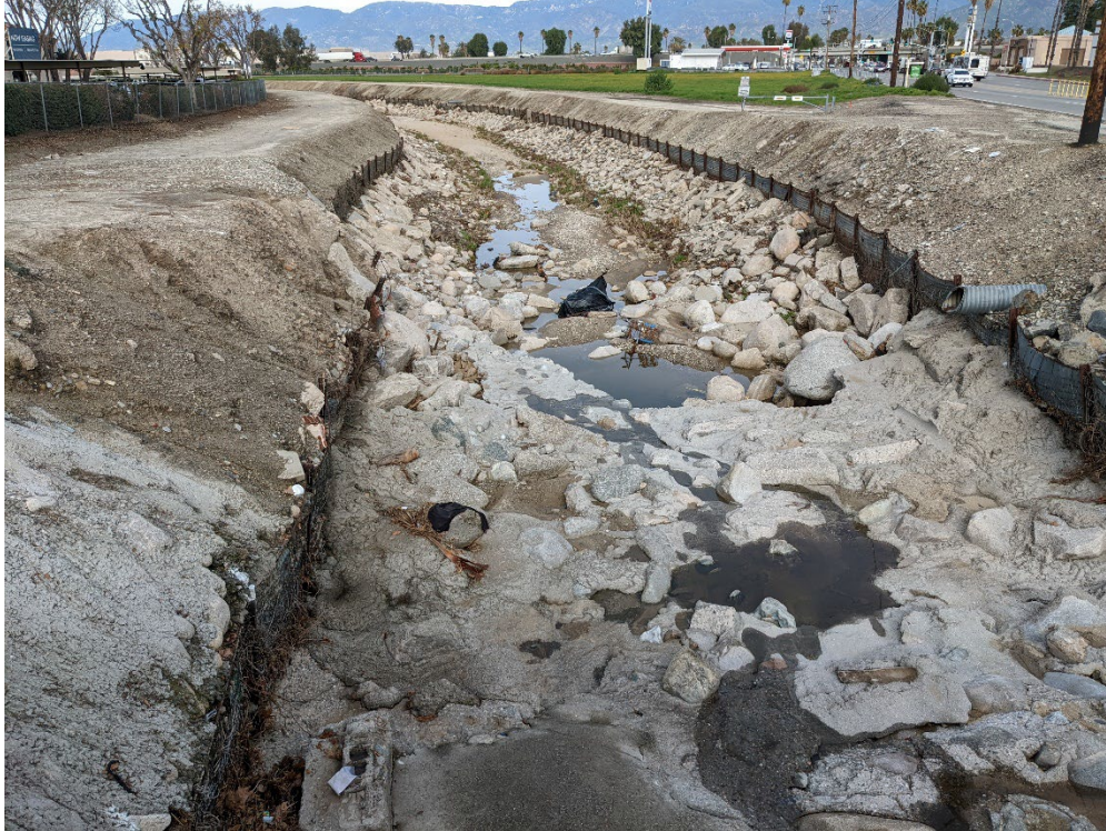
Figure 6. Overview of Mission Creek Channel looking northwest.
