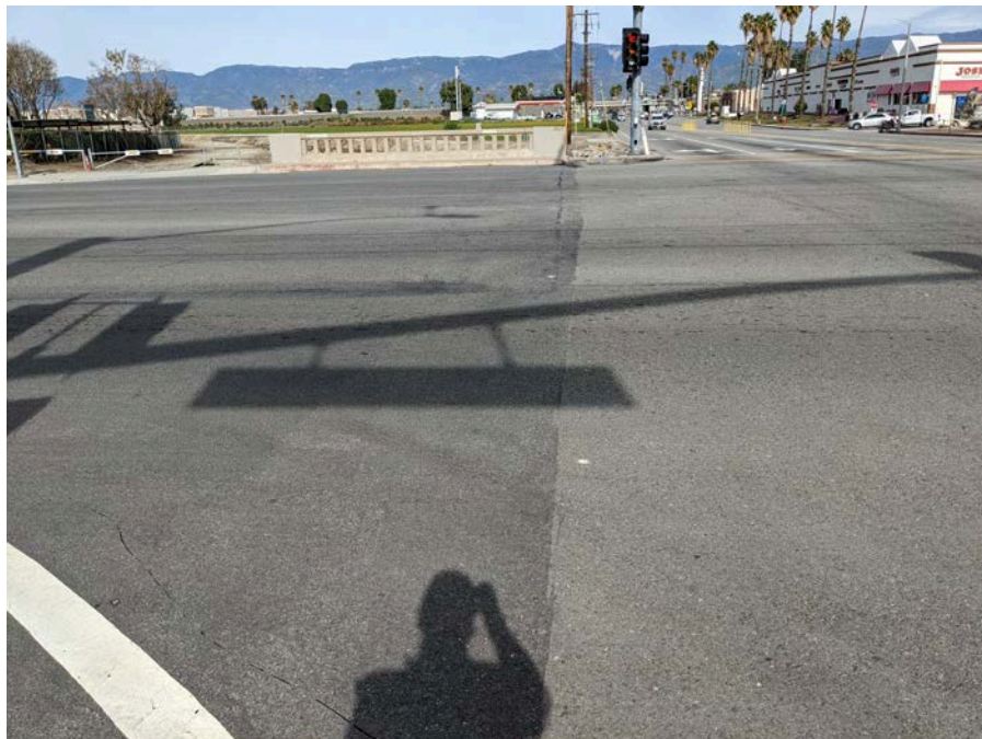
Photograph 6: View looking north across Redlands Boulevard at the remaining concrete railing over the Mission Creek Channel.
