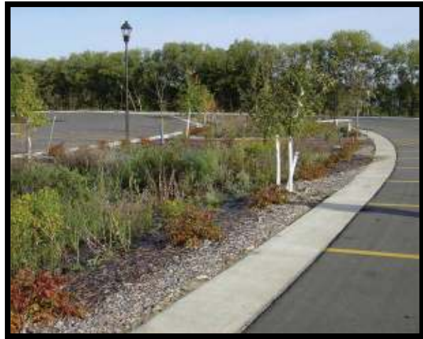
Vegetated swale with a zero-curb used as a parking lot planter.
