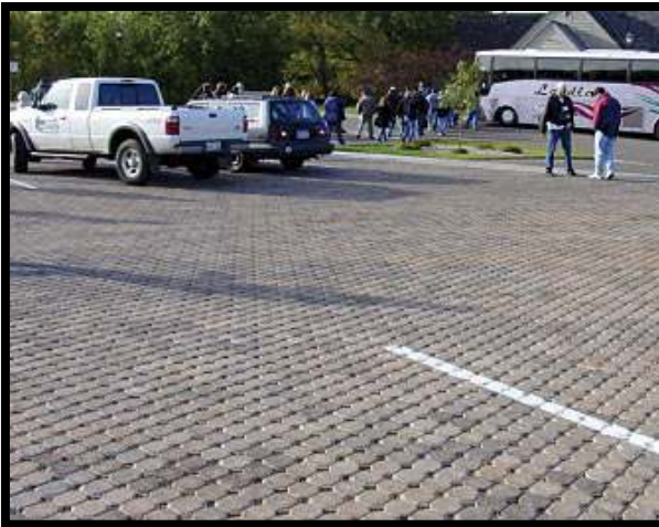
Permeable paving used for parking stalls.
