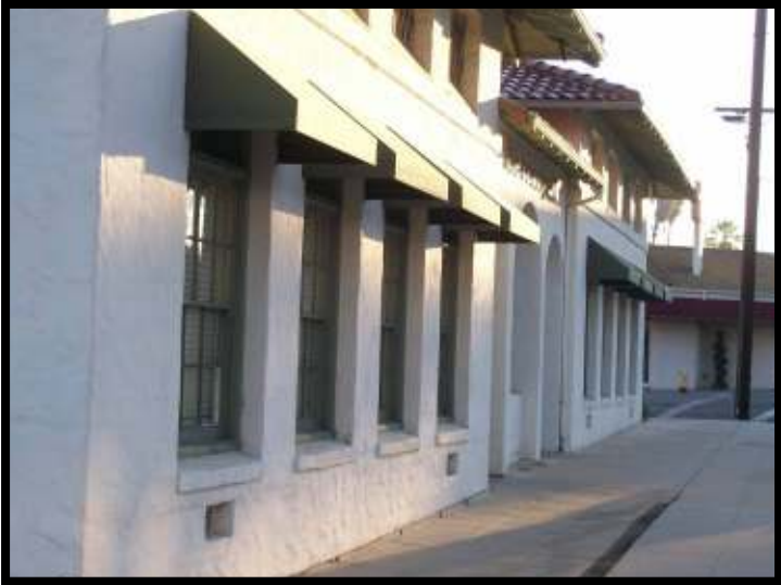
Windows can either be recessed or project out from the building surface to provide depth to building elevations.
