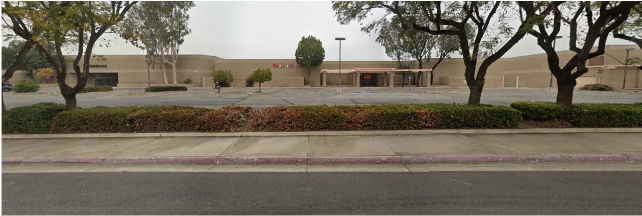
Existing views looking north towards the Project Site from W Citrus Avenue.
