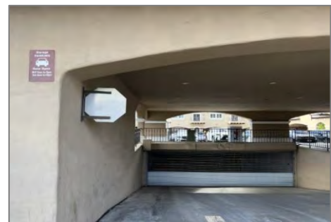
Entrance to Centennial Plaza Garage
