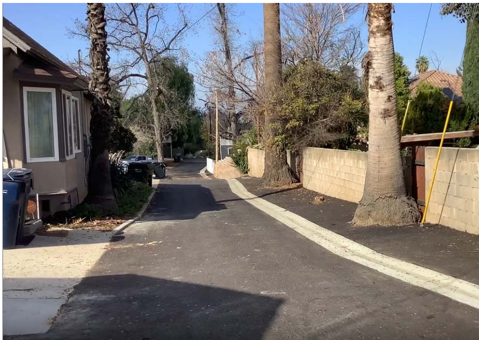
Alley Repaving Project – before and after on Steele Street
